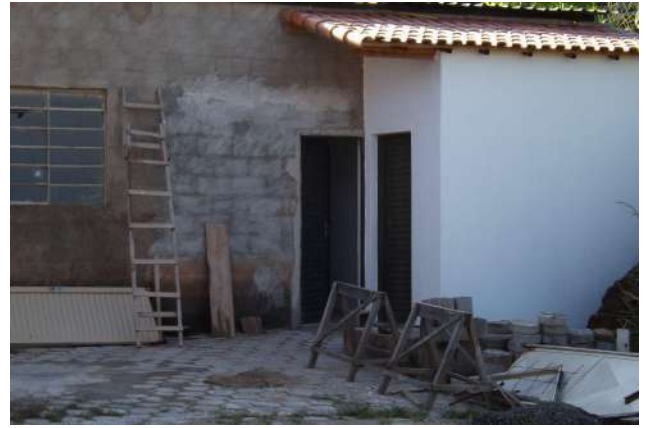
Figure 12: Machado Campus improvements in the Mechanization Sector
