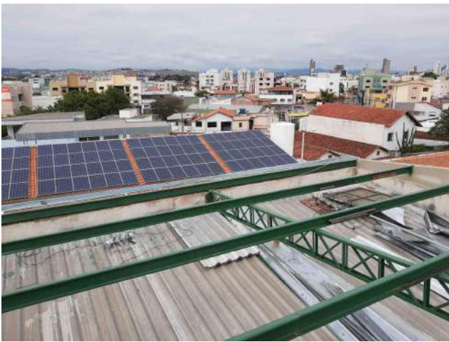
Figure 27: Rectory roof renovation.
