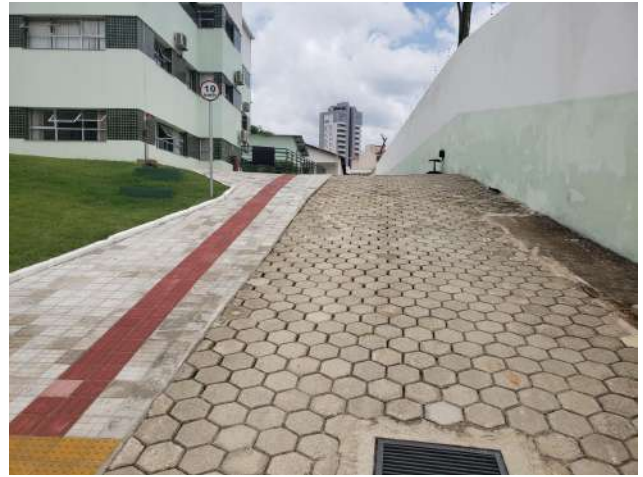
Figure 30: Rectory renovation of the drainage system.
