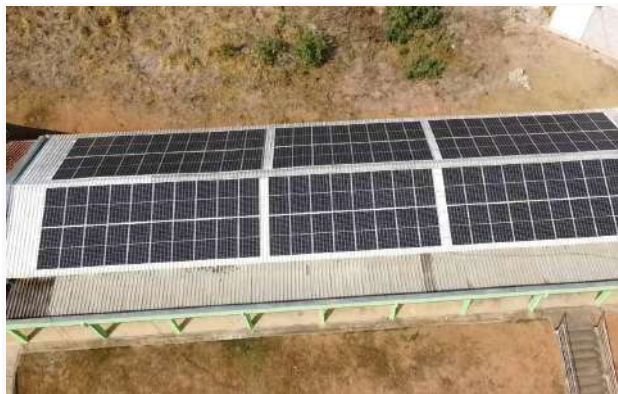
Figure 21: Machado Campus implementation of new photovoltaic modules.
