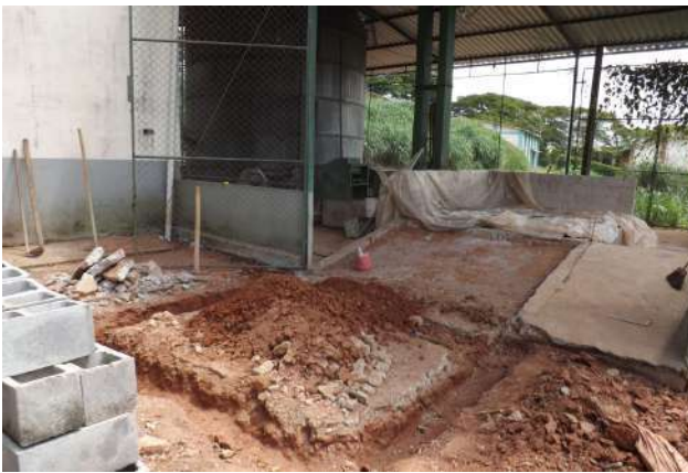
Figure 13: Machado Campus Feed Factory improvements.
