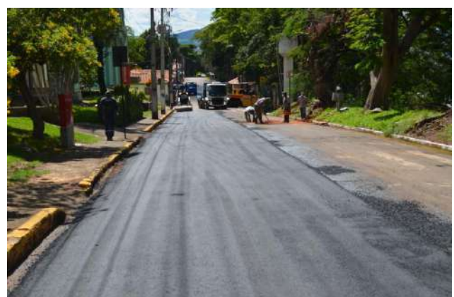
Figure 4: Machado Campus street paving refurbishment.
