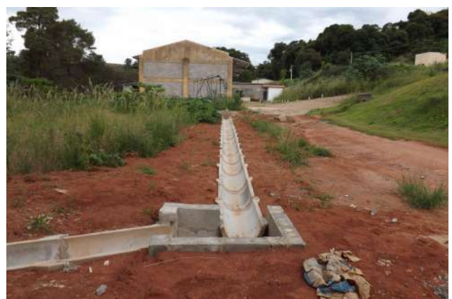
Figure 8: Machado Campus streets drainage.
