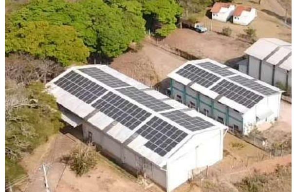
Figure 22: Machado Campus implementation of new photovoltaic modules.
