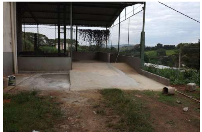
Figure 14: Machado Campus Feed Factory improvements.
