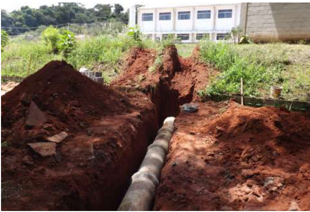
Figure 7: Machado Campus streets drainage.
