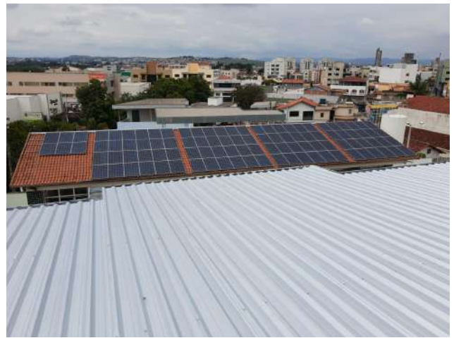
Figure 28: Rectory roof renovation.
