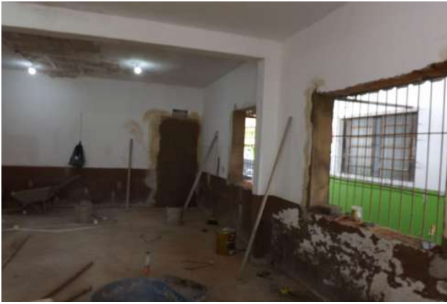
Figure 5: Machado Campus renovation of the Nursing Laboratory.
