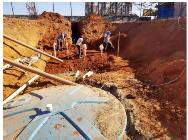
Figure 20: Machado Campus implementation of the Sewage treatment system of the Coffee Center of Excellence.
