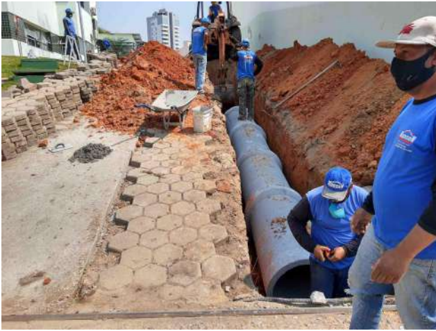
Figure 29: Rectory renovation of the drainage system.
