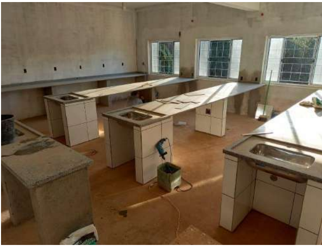
Figure 35: Inconfidentes Campus renovation of the Environmental Laboratory.
