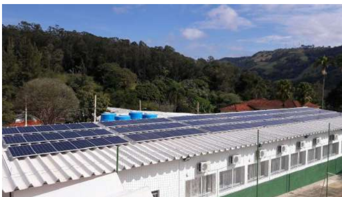
Figure 7: Campus Carmo de Minas solar power plant.
