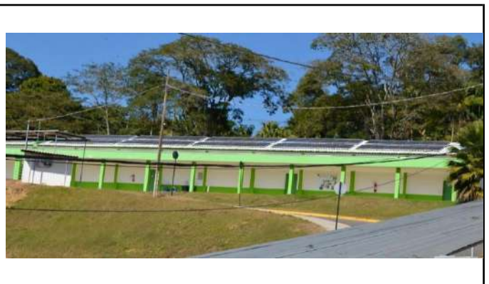
Figure 2: Campus Machado solar power plant.
