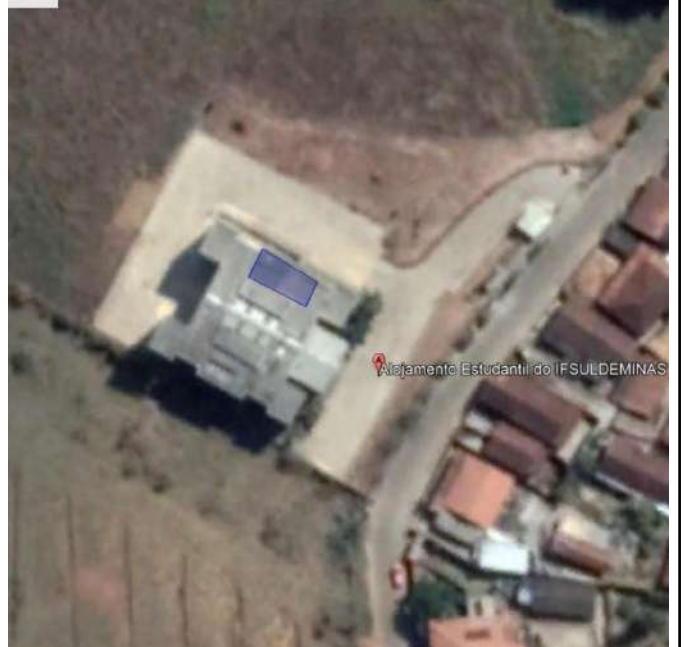
Figure 16. Inconfidentes Campus Solar water heating system.
