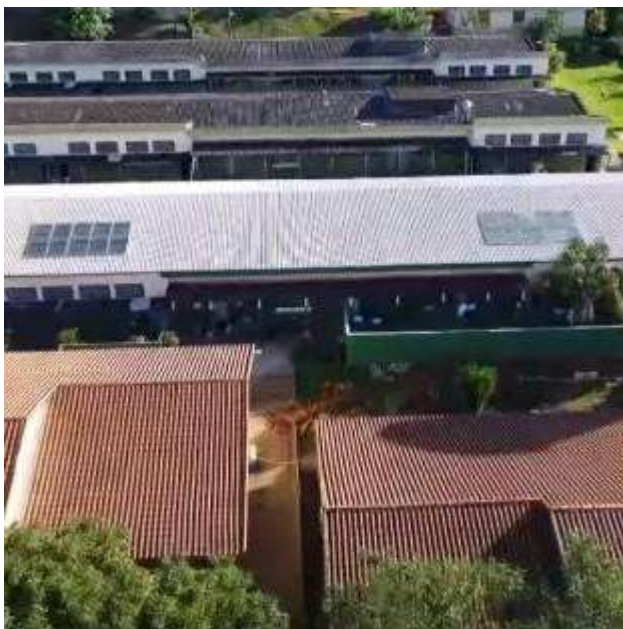
Figure 15. Inconfidentes Campus Solar water heating system.
