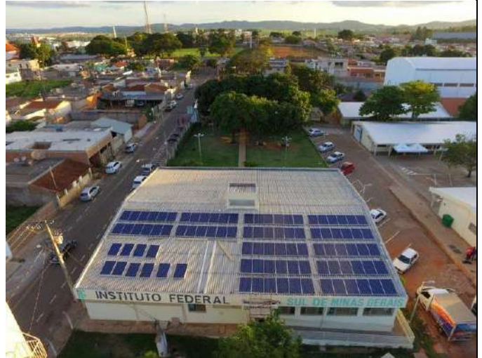
Figure 4: Campus Passos solar power plant.
