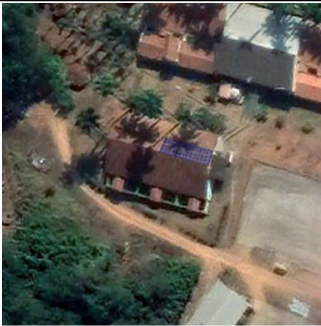
Figure 17. Machado Campus Solar water heating system.
