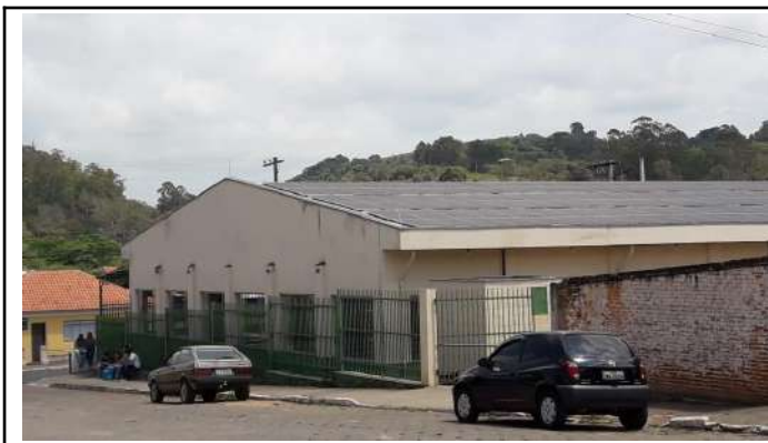
Figure 1: Campus Inconfidentes solar power plant.
