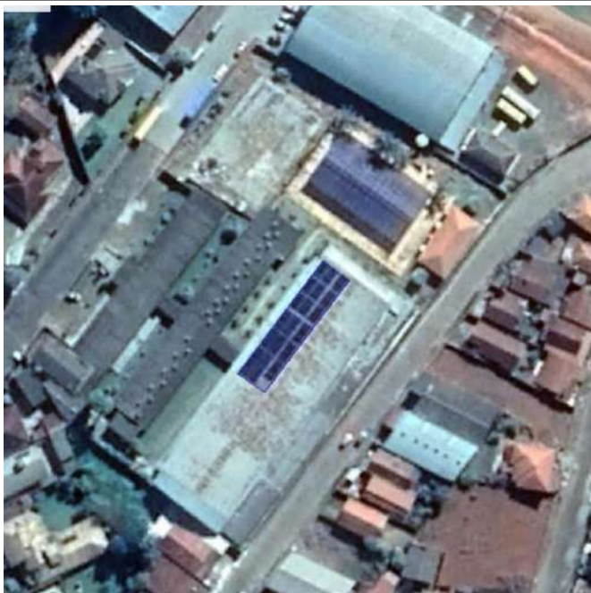
Figure 19. Muzambinho Campus CeCAES Solar water heating system.
