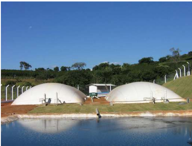
Figure 13. Swine waste treatment unit for biogas production.
