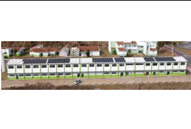
Figure 21 : Campus Machado expansion of the photovoltaic plant.
