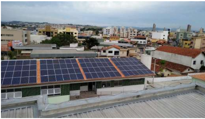
Figure 9: Rectory solar power plant.
