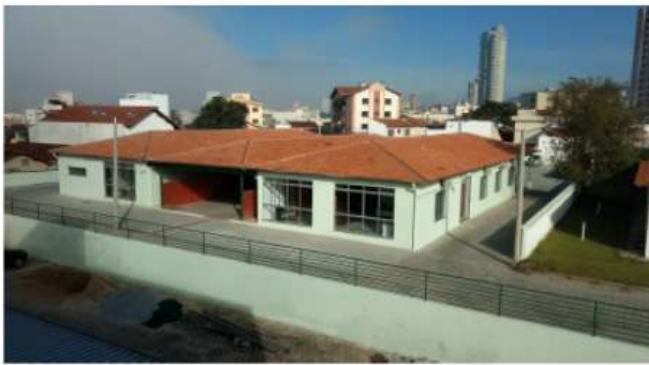
Figure 1: Rectory natural ventilation and lighting
