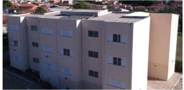
Figure 26: Inconfidentes Campus Visconde de Mauá student building solar heating system.
