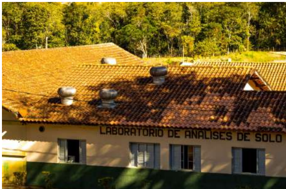
Figure 19: Campus Inconfidentes Soil Analysis Laboratory exhausters.
