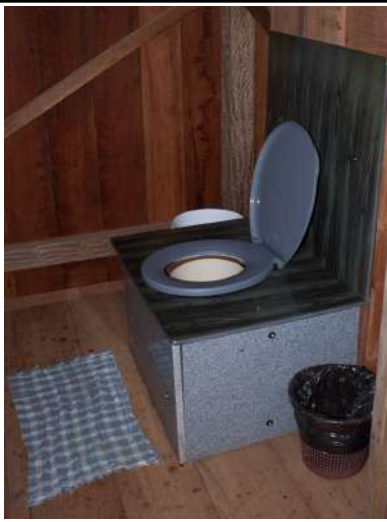
Figure 23: Inconfidentes Campus dry toilet at Agroecology Sector.
