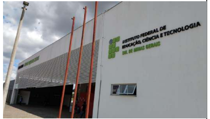
Figure 20: Campus Poços de Caldas building facade brise-soleil.
