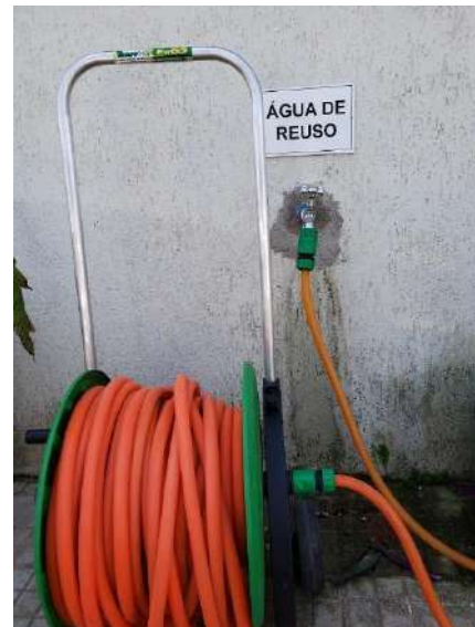
Figure 18: Rectory sign indicating reused water tap.
