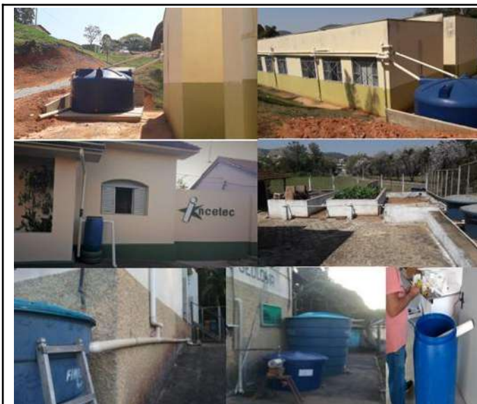
Figure 1: Campus Inconfidentes rain harvesting system.
