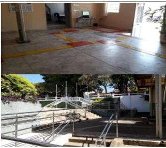
Figure 8: Inconfidentes Campus tactile paving, ramp and handrails.
