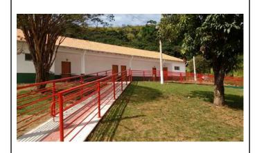
Figure 5: Carmo de Minas Campus tactile paving and handrails.
