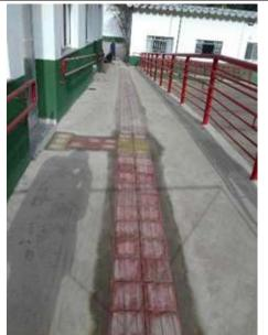
Figure 4: Carmo de Minas Campus tactile paving and handrails.
