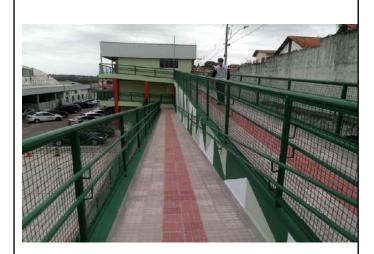
Figure 9: Três Corações Campus tactile paving, ramp and handrails.
