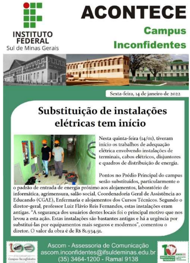
Figure 22: Inconfidentes Campus replacement of electrical installations.
