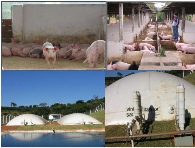
Figure 11: Muzambinho Campus swine waste treatment.
