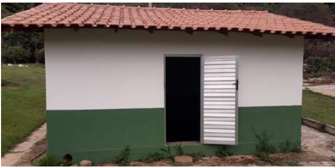
Figure 20: Carmo de Minas Campus water storage cisterns with a capacity of 80,000 liters.
