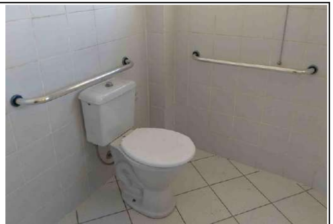
Figure 2: Rectory toilet water box flush.
